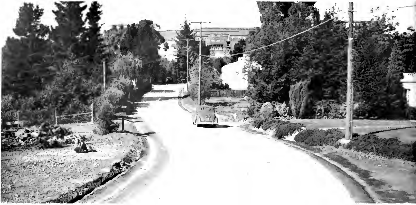
Alameda Access Road to San Leandro Naval Hospital in Oakland. View shows concrete pavement on heavy grade. Hospital building in background
